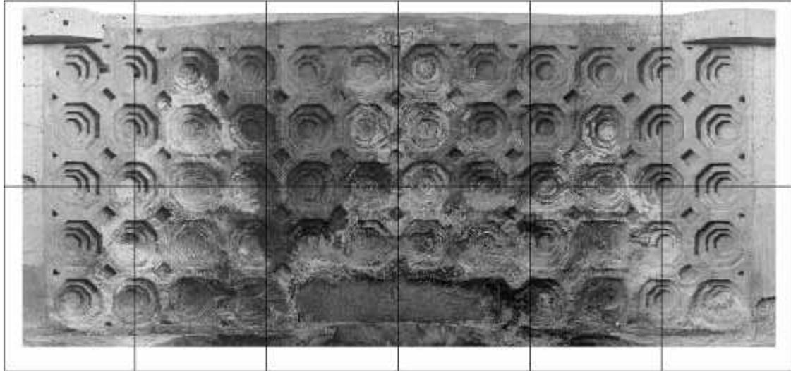
Fig. 12: Image map of the unwrapped middle vault
