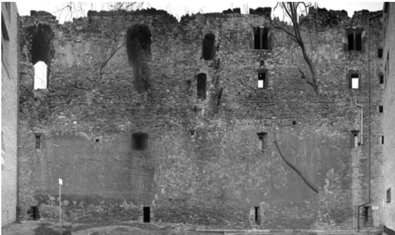
Figure 7: Digital unwrapped image mosaic of the West-Tower of the Moritzburg, Halle
