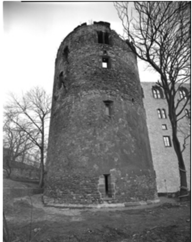
Figure 6: Metric photograph of the West-Tower of the Moritzburg, Halle
