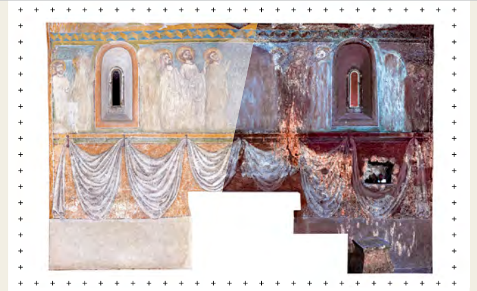
Castle Katzenstein, Chapel True to scale unwrapping of the apse with ortho projection, congruent superimposition of colour image (left) and UV-light image
